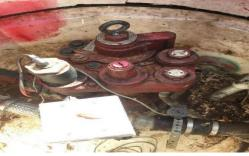
The fuel station Veeder-Root monitoring and safety control system is antiquated technology, this includes the leak detection system and automated valves. Repair parts and materials are becoming increasingly obsolete, limiting maintenance options. Underground piping and plumbing
